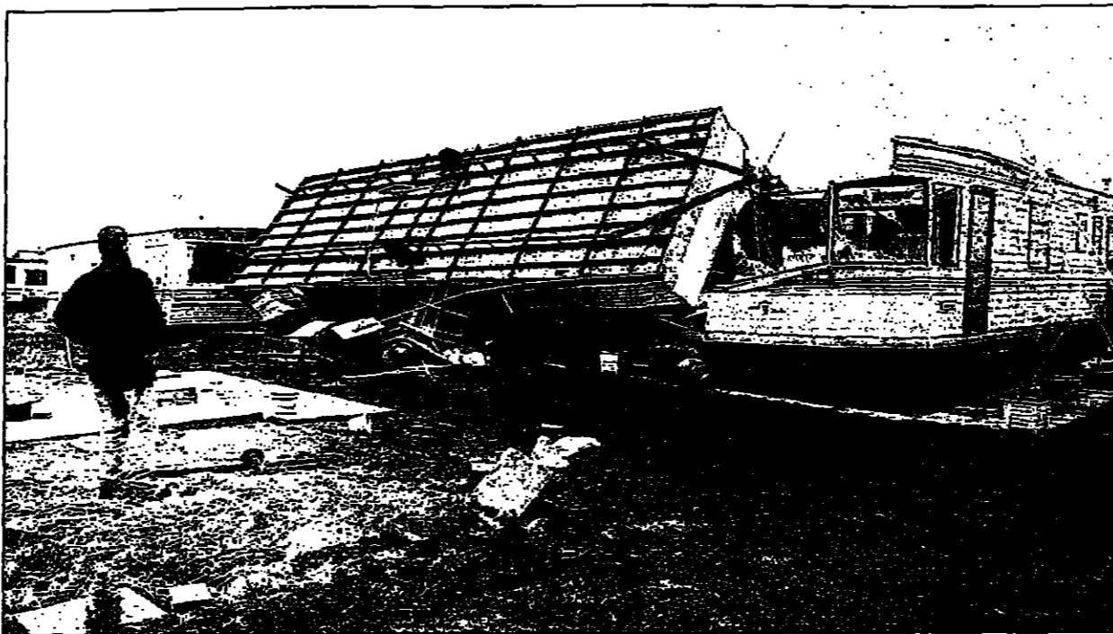
Premiums may rise if bad weather continues to cause damage to property, such as caravans on this site in Northumberland
